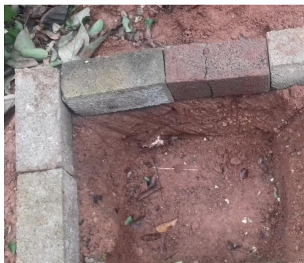
MAN – MADE COMPOST PIT (4X3X2 Ft) THE FOR DISPOSAL OF BIO DEGRADABLE WASTE
