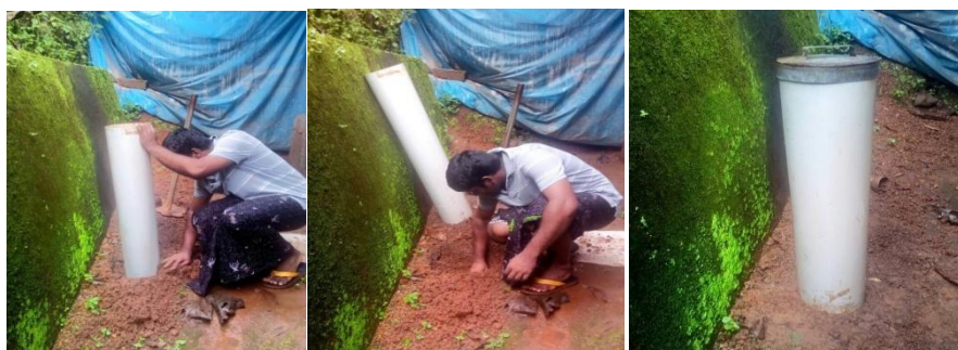
Installing Pipe compost
